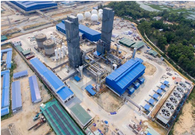
Air separation units under construction in Dung Quat, Vietnam
